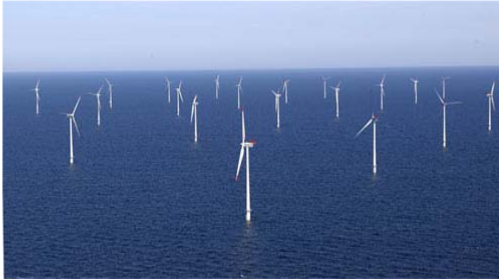
Fig. 4. Horns Rev offshore wind farm, Denmark [21]
