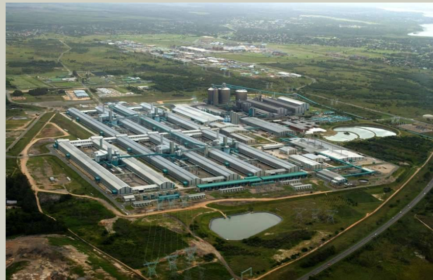
BHP Billiton's Hillside Smelter, Richards Bay, South Africa
