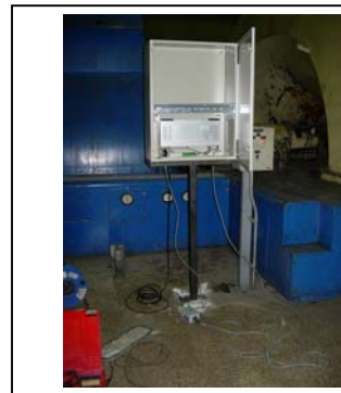
Image 3- Telemetry receiver installed into a box
