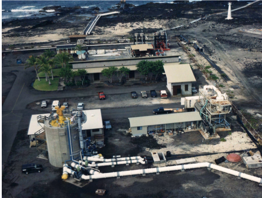
Figure 16.3: 210kW OC-OTEC Experimental Plant (1993-1998) in Hawaii
