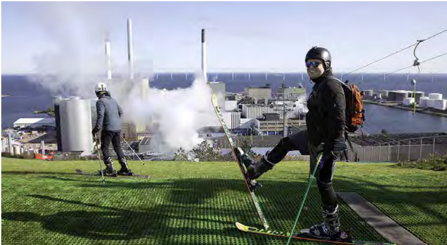
Copenhill illustrates a different urban approach by integrating essential energy infrastructure directly into the city. Credit: Max Mestour and Amelie Louys.
