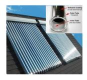
b) Evacuated tube collectors (inset: tube used)
